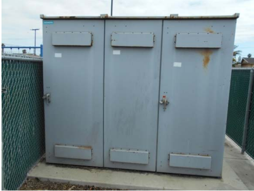
Photo #37: Main Electric Switchgear Box
