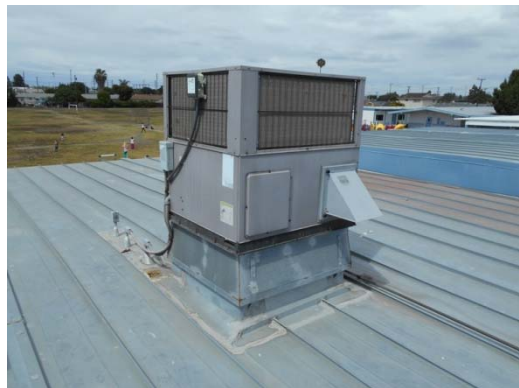
Photo #30: Roof Mounted Heat Pump
