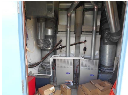
Photo #28: Split System Air Conditioning Furnaces
