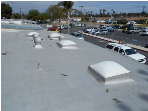
Photo #21: Built-up Roof with Skylights
