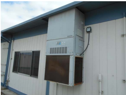
Photo #29: Wall Mounted Heat Pump
