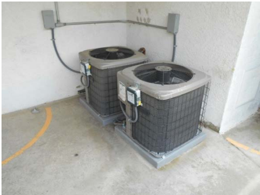
Photo #27: Split System Air Conditioning Condensing Units
