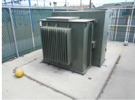
Photo #38: Pad Mounted Transformer
