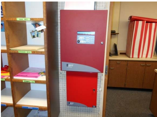
Photo #35: Central Fire Alarm Panel
