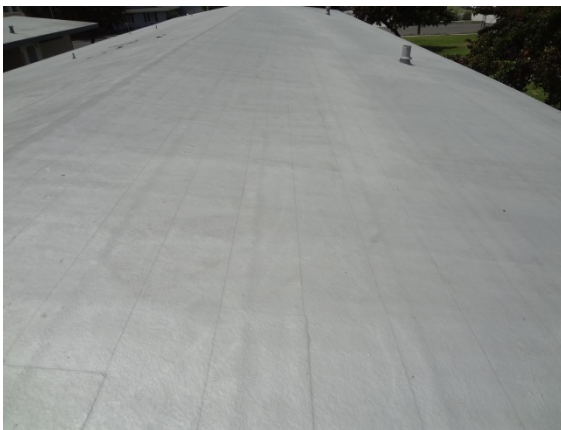
Photo #17: Asphalt Membrane Roofing
