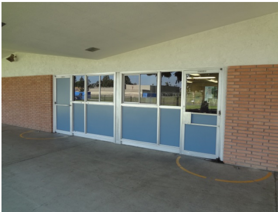
Photo #23: Administration Building Exterior Doors and Single Pane Fixed Windows
