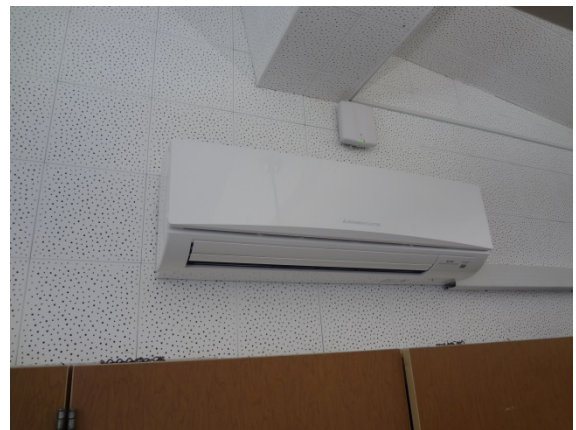
Photo #30: Ductless Split System Evaporator
