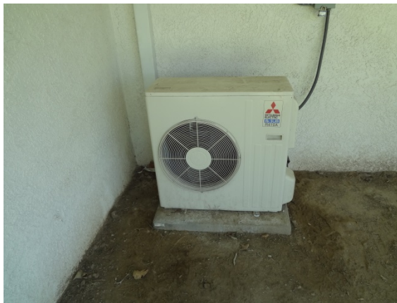
Photo #33: Ductless Split System Condensing Unit
