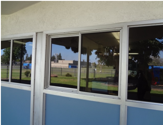
Photo #21: Single Pane Slider Window
