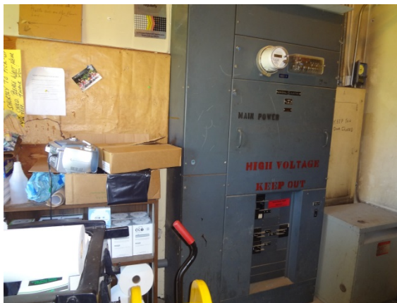
Photo #47: Main Switchboard
