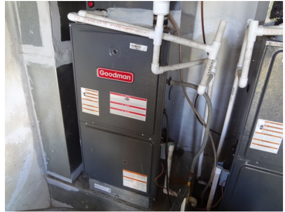
Photo #44: Newer Gas Furnace
