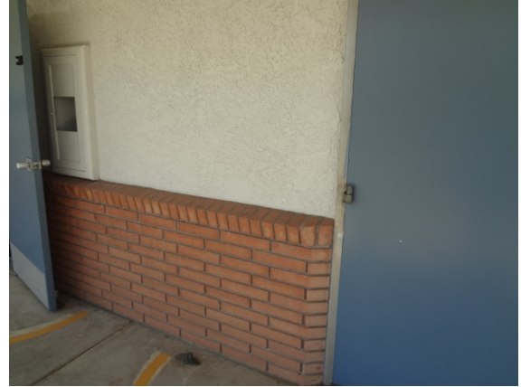
Photo #20: Building Façade Brick Veneer and Stucco
