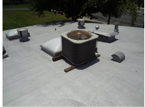
Photo #26: Administration Building Condensing Unit
