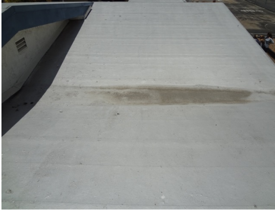
Photo #19: Low Point with Potentially Ponding Issues
