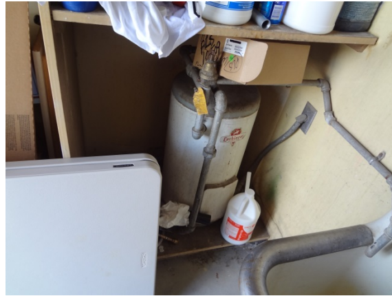
Photo #38: Failed Electric Water Heater
