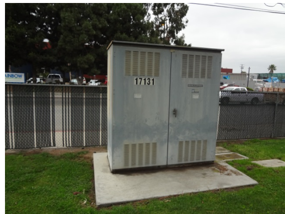
Photo #30: Main Service/Switchboard (Utility Company Managed)
