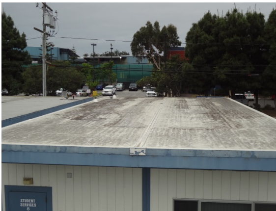
Photo #15: Room 8 Single Ply Membrane Roof
