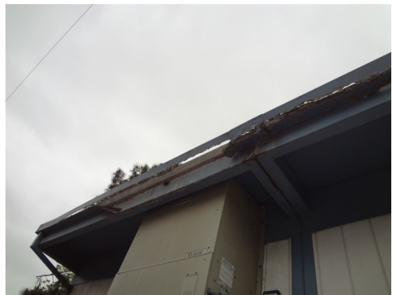
Photo #18: Corroding Structural Members and Gutter System Room 9
