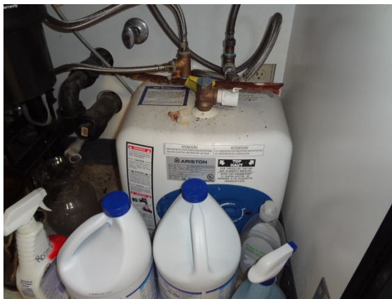
Photo #29: Office Point of Use Electric Water Heater
