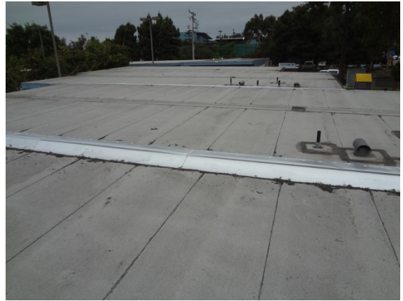
Photo #14: Asphalt Membrane Roof
