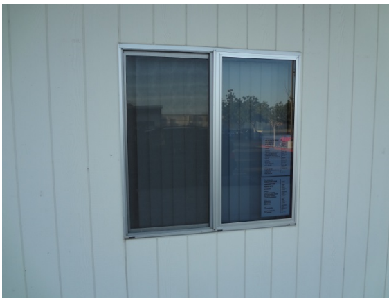
Photo #17: Engineered Wood Siding and Double Pane Slider Style Window
