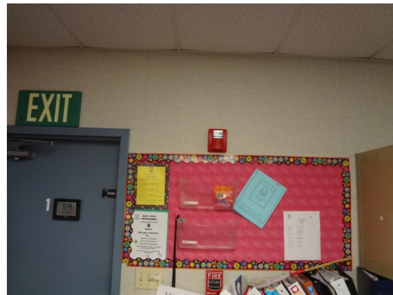
Photo #22: Fire Alarm Device and Illuminated Exit Sign
