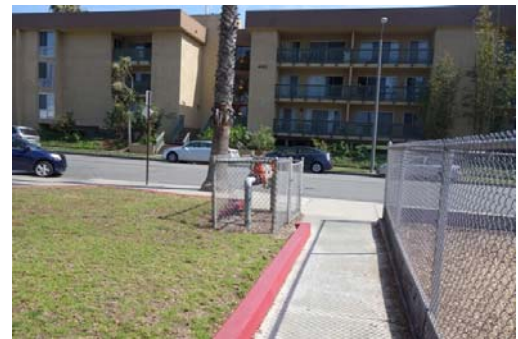
Photo #22: Main Water and Back Flow
