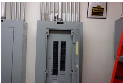
Photo #27: Sub Panel Circuit Breaker Panel
