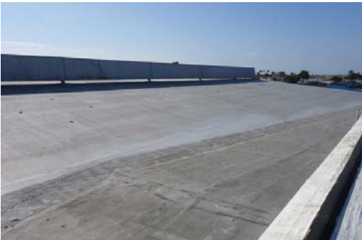
Photo #58: Older Builtup with Elastomeric Spray
