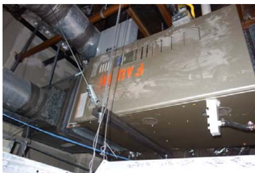
Photo #54: Ceiling Coil and Furnace on East Section
