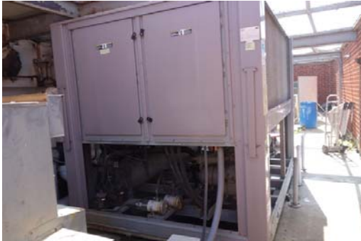
Photo #31: Carrier Air Cooled Chiller
