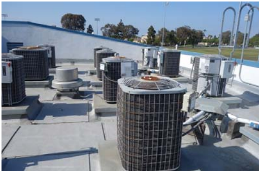
Photo #55: Roof Mounted Split Unit Compressors for East Section
