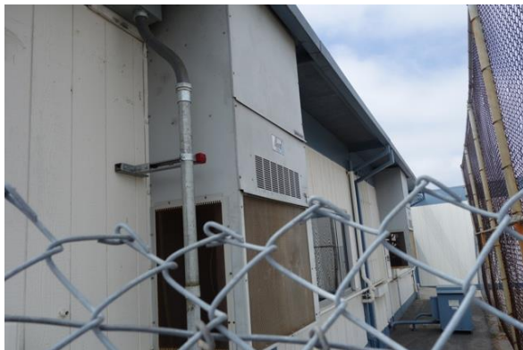
Photo #57: Wall mounted package unit for Pod
