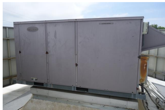
Photo #59: Carrier RTU – 25 Ton (typical)
