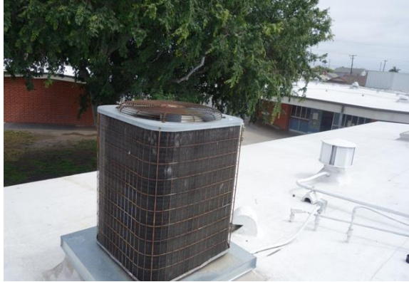
Photo #49: Admin Building Condensing Unit
