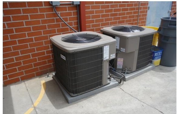
Photo #4: MPR Split Unit Condensers
