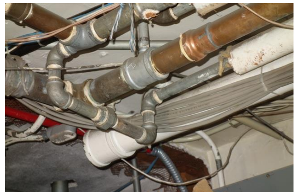
Photo #12: Copper and Galvanized Domestic Water Piping
