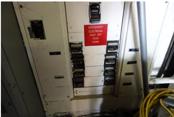
Photo #9: Electrical Main Disconnect
