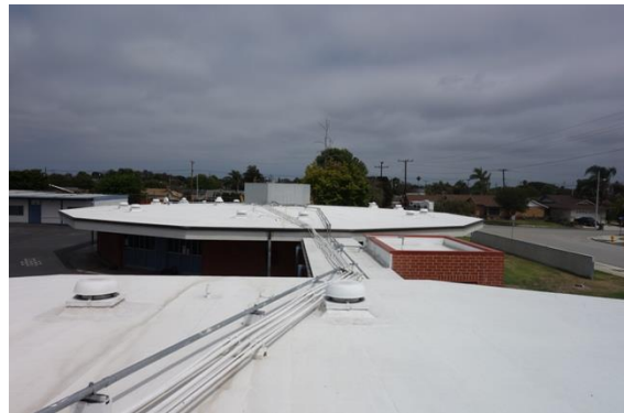
Photo #60: Elastomeric Roof Coating (typical)
